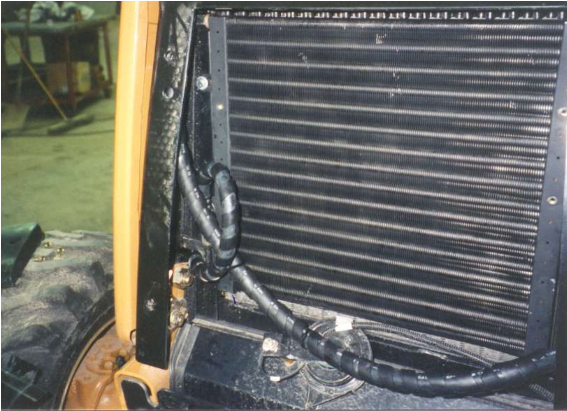
Condenser mounted with hoses in place.
