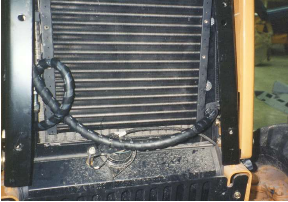
Condenser in place showing hose routing.
